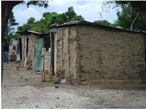
House with clissage 20 walls and plain roof probably wooden boards or tin planks 21
