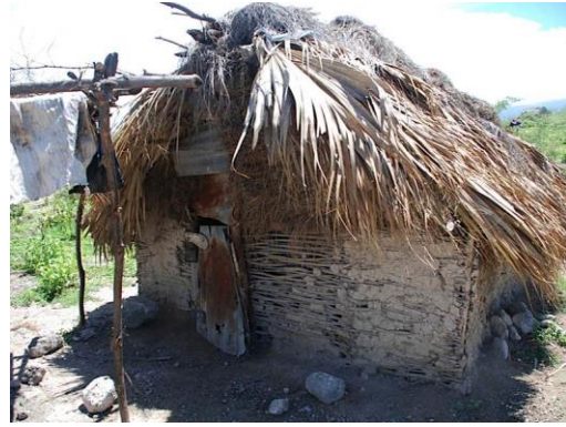
House with earthen walls and palm leaves double gable roof 22
