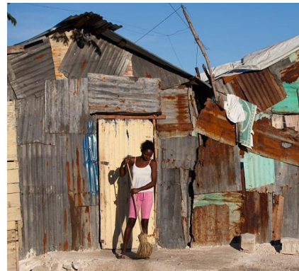
Slum house made of pieces of tin planks 24
